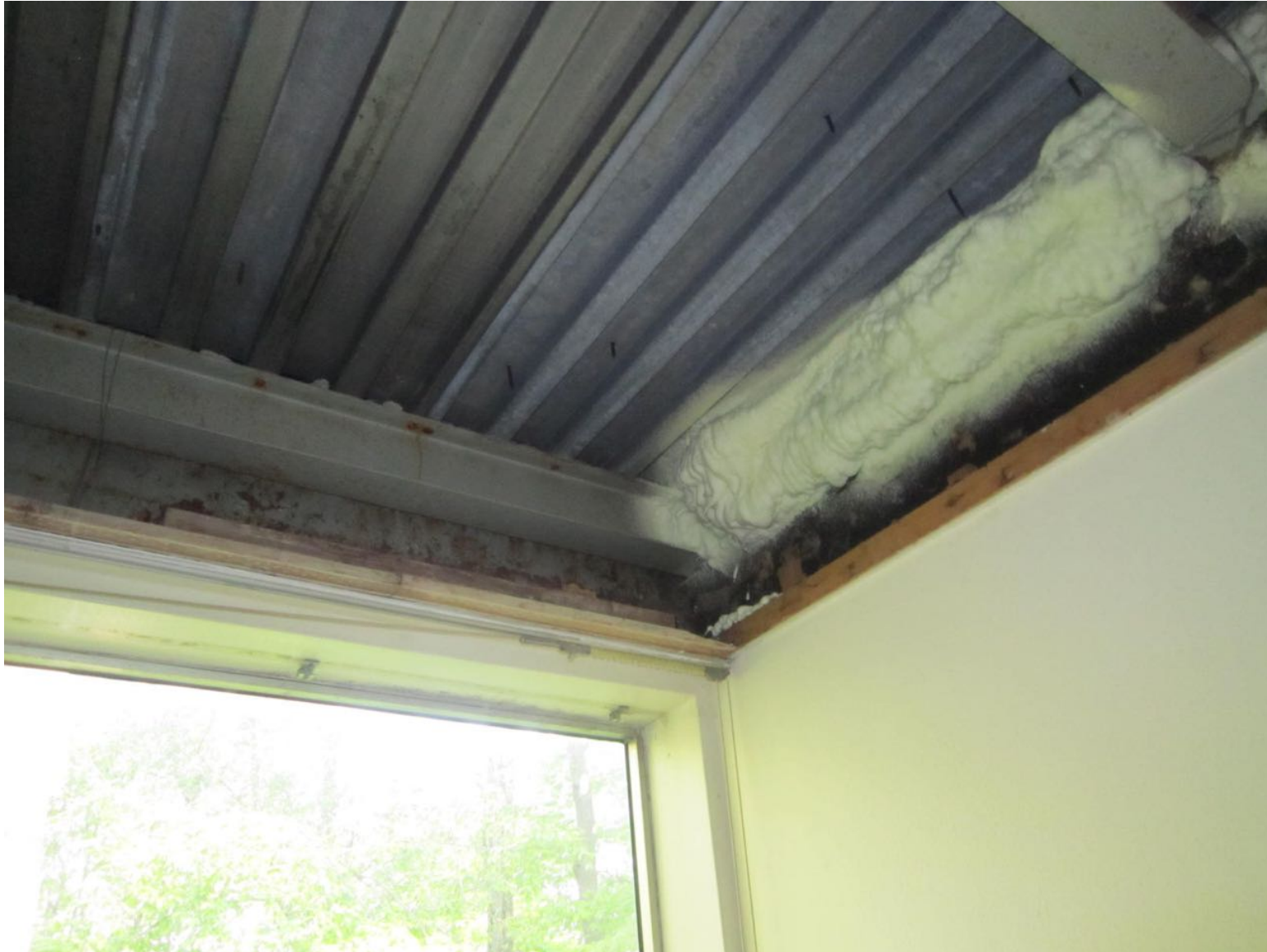
Chapel House- Construction – Airsealing
