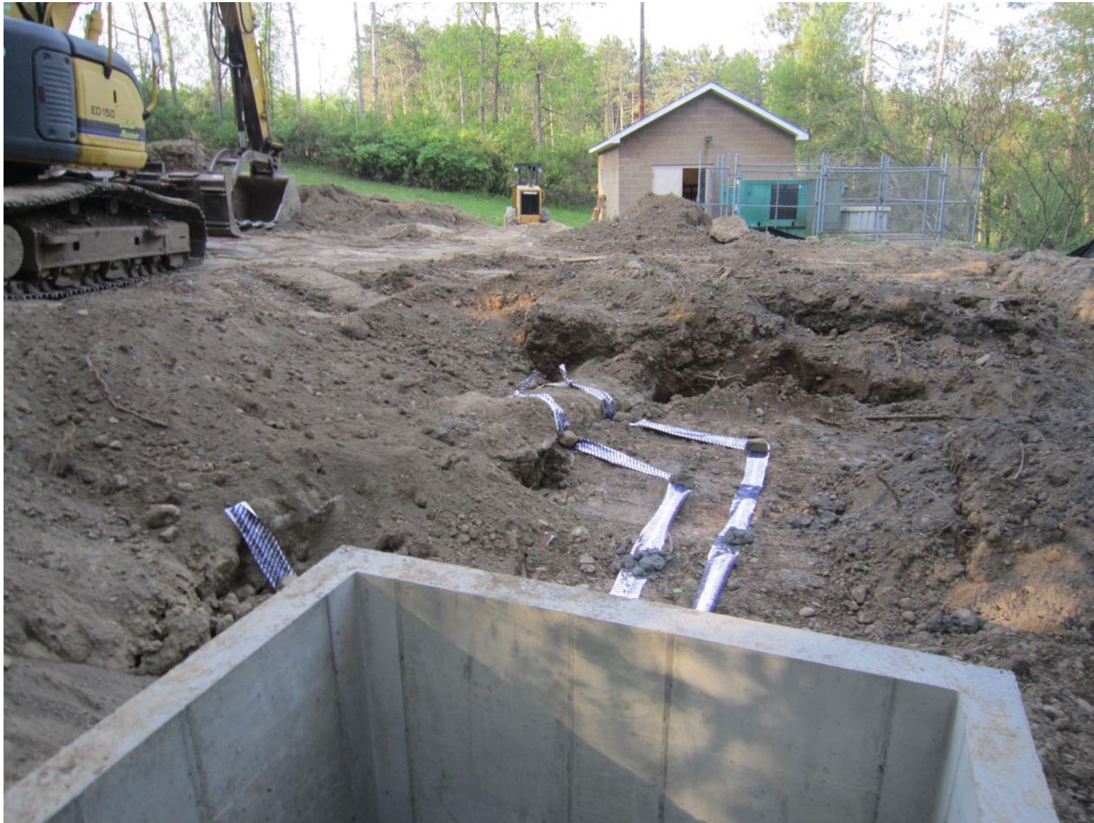
Chapel House- Construction – Geo well vault
