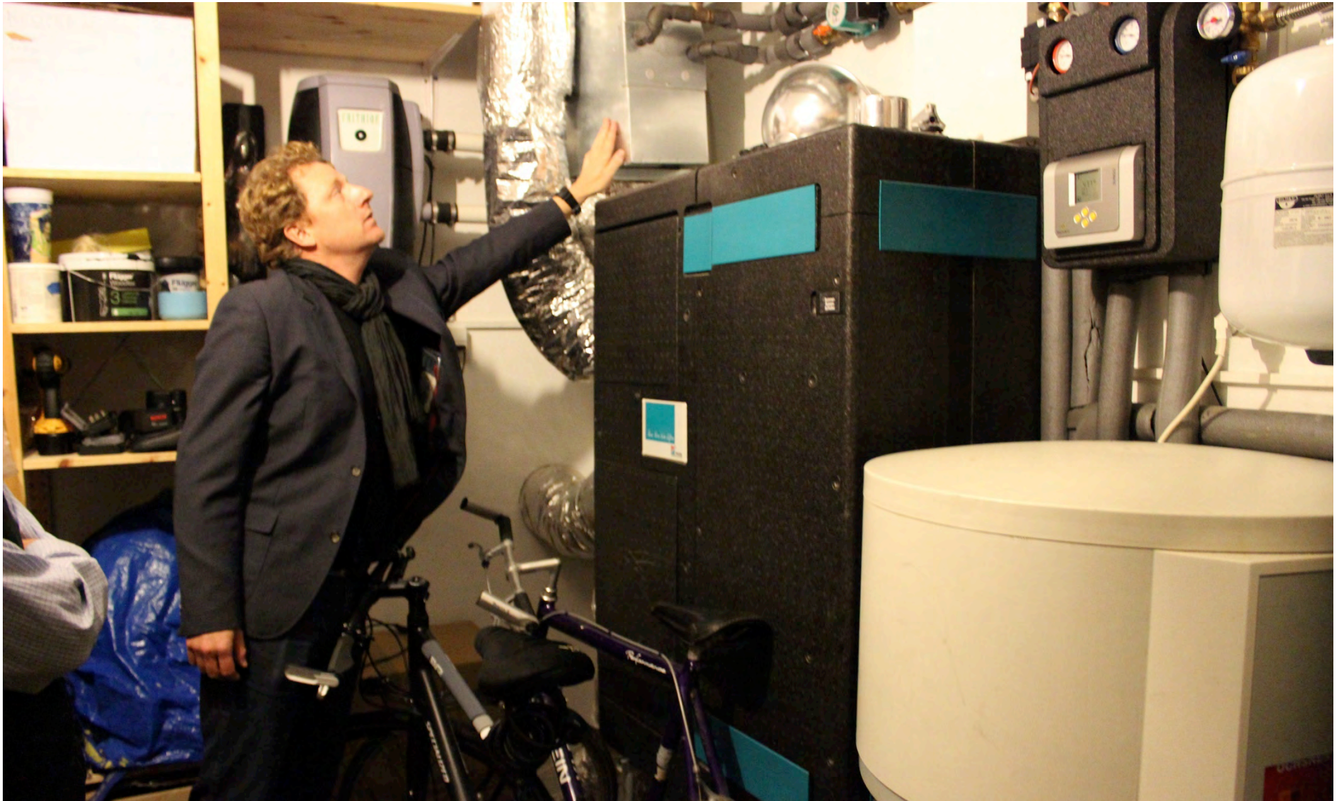
Mechanical Systems- Heat pump and ERV with ground pre-heat
